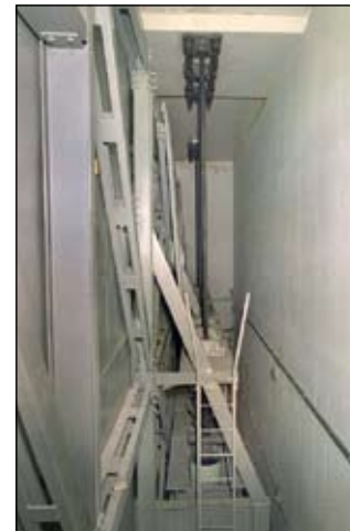
Plate 11 - Honecker's bunker, internal image showing a 'bunker within a bunker' the inner structure is suspended from springs within an outer underground shell
